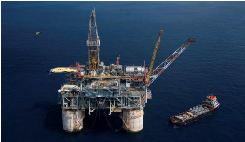
Supplying More Natural Gas
