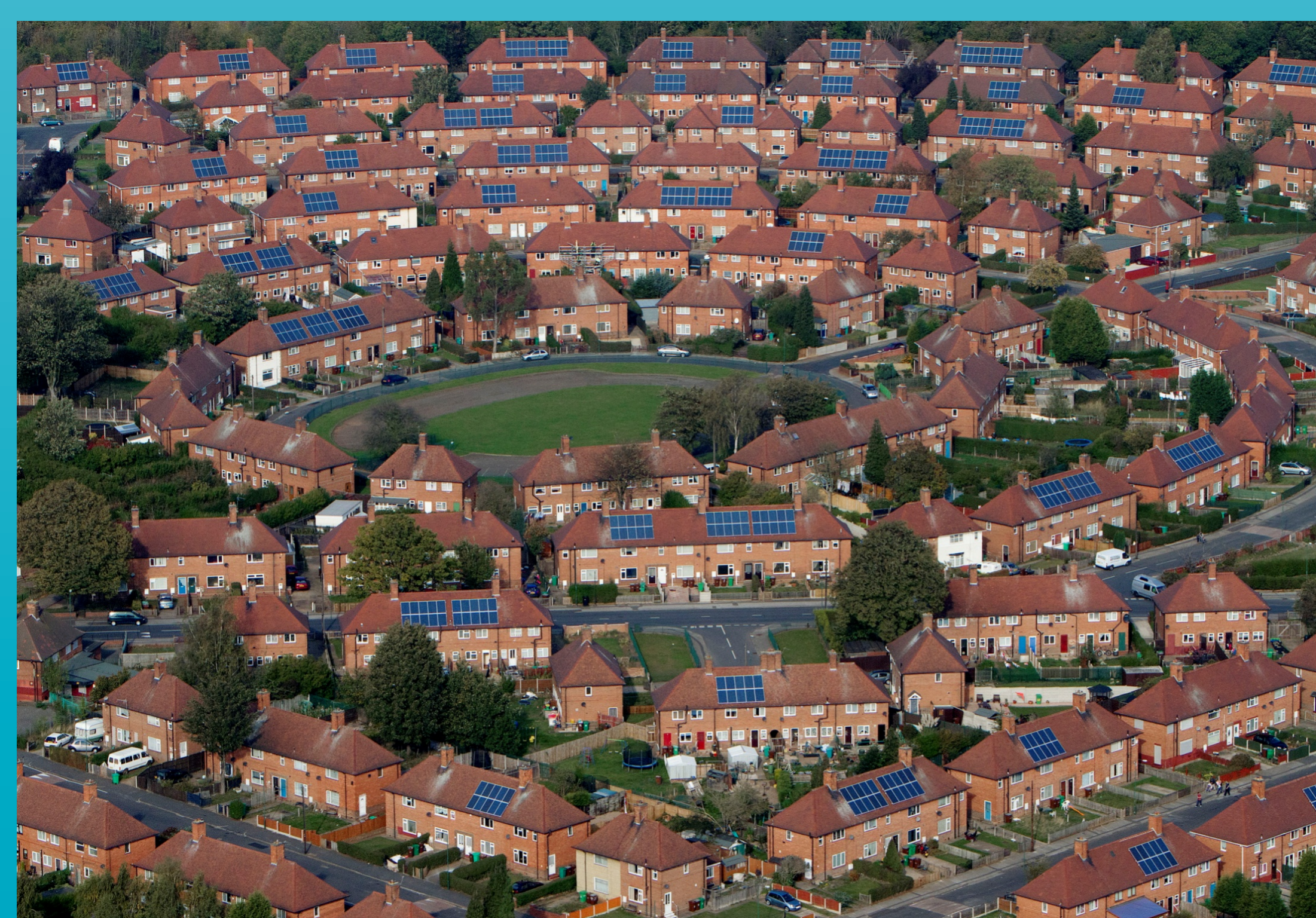
Source: E.ON Sustainable Energy
